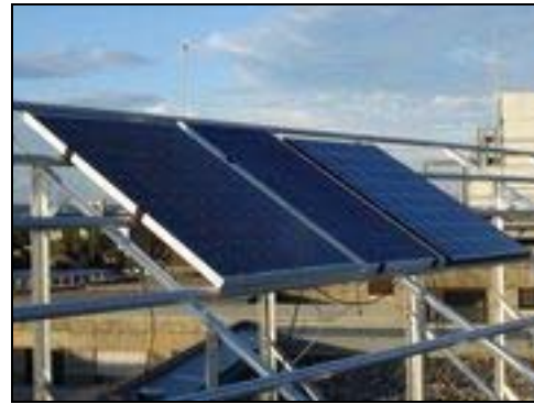
Figure 5: Installation of three different PV modules: mono-Si, multi-layer a-Si and poly-Si
